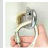
**3** Check installation by tugging the eyebolt. In the secure position, the word "LOCKED" is fully visible on the trigger. A safety lanyard attached to a full-body harness can now be connected to the eyebolt—and the user can begin working.
